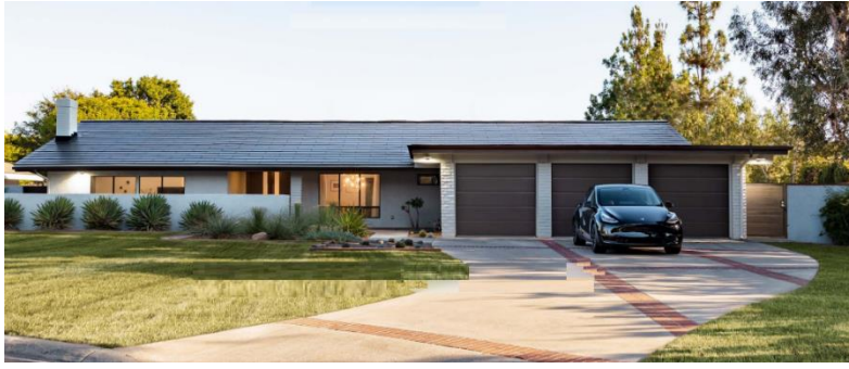
Figure 1 – Solar Roof. Produce clean energy from roof
