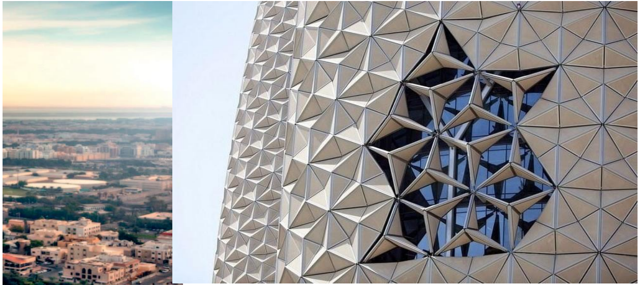
Figure 1 – Fast-responsive building components
